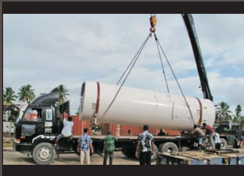
Equipment for Government Dept. To be relocated to Labasa
