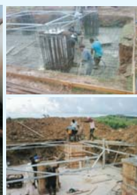
Hi-tech Rigging Limited A local company contracted to build the majority of Vodafone /Digicel /Fintel Towers around Fiji Islands and lately given the contract at PNG for Digicel. 100% Standard Concrete Industries Client. Pictures from Natadola Vodafone Tower site 110m3 was poured for this site.
