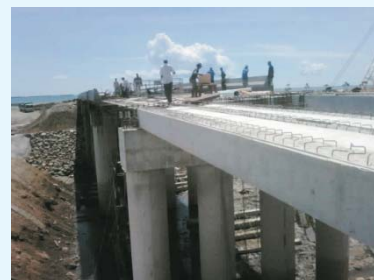
Naisoso Bridge: Herbert Construction project Supplied by SCI
