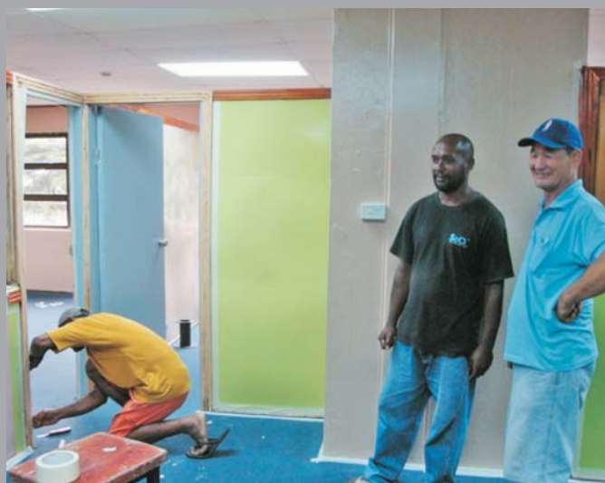
PMO (Levani) supervising construction works for Vanua House tenant.
