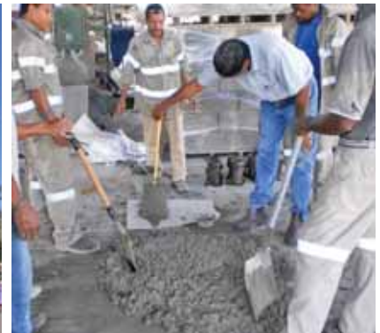
Mixing of concrete for test cylinders using Pacific cement at PNG Ready Mix.
